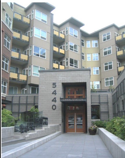
Acceptable concrete block use/design.
